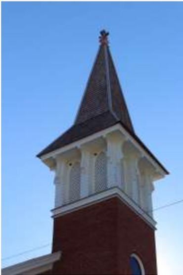
Above: The belfry roof was replaced with wood shingles, the lattice and metal screen were repaired, and the finial was replaced. Interior work included installation of structural steel.
