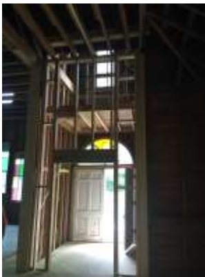
Left and right: Necessary repairs were made to the interior framing to restore the building's structural integrity.
