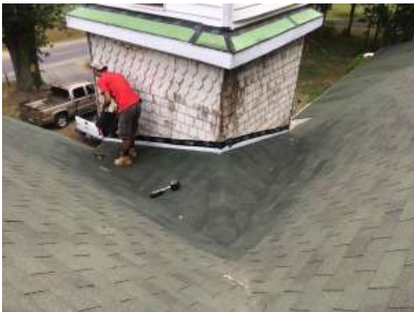
Above: repairs to roof cricket above bell tower to prevent continued water intrusion.
