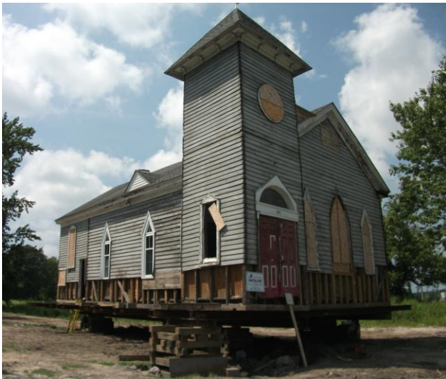
Above: Church during lifting and foundation repairs phase in the fall of 2012.
